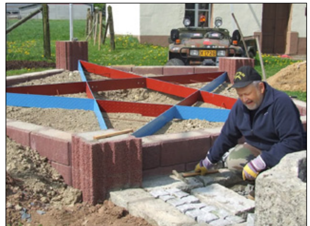
Norbert shown building the new monument.
